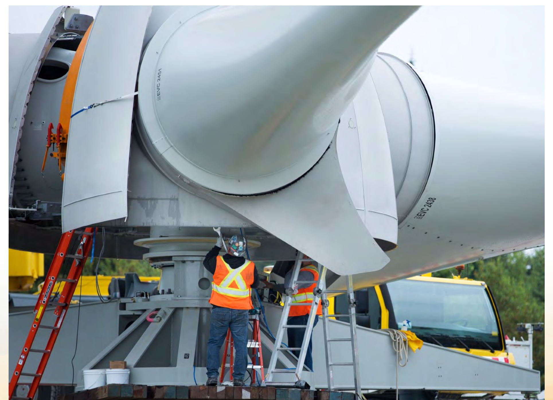
Staff working during the assembling of a turbine. Québec
